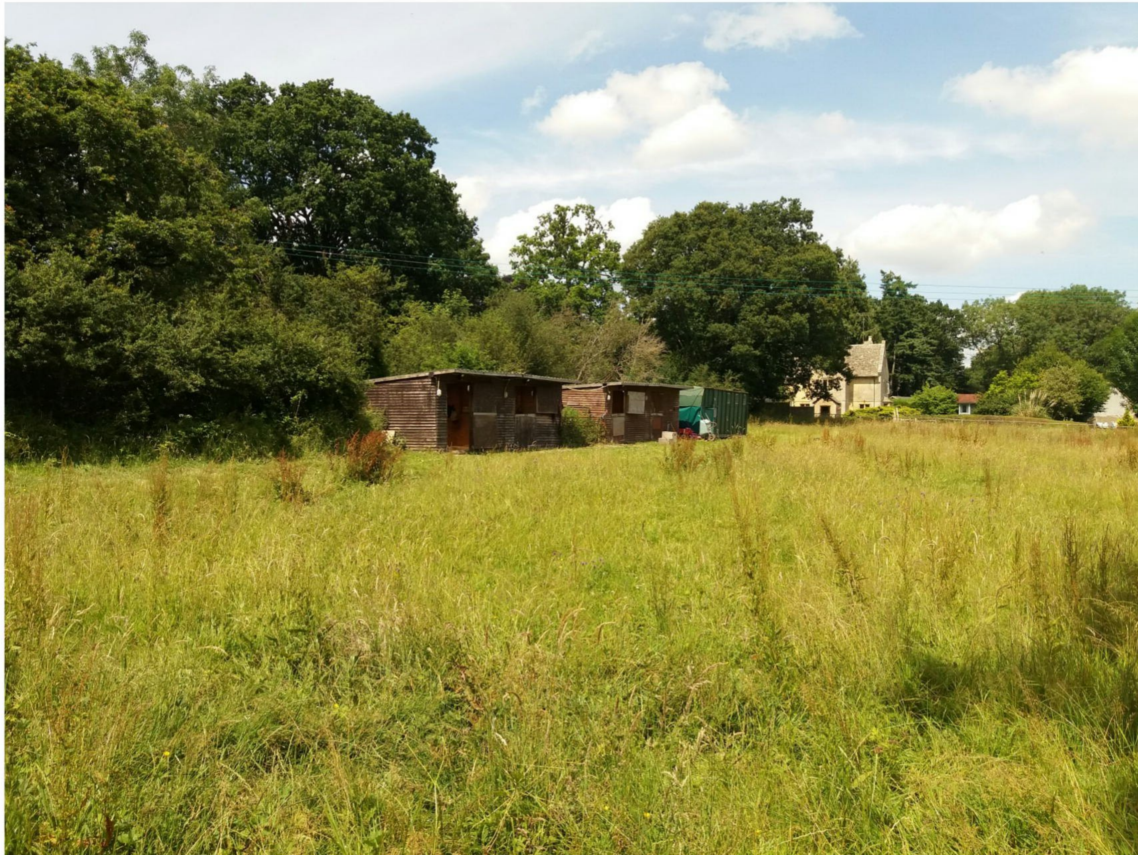
3. Stables off Greenway Lane adjacent to public footpath
